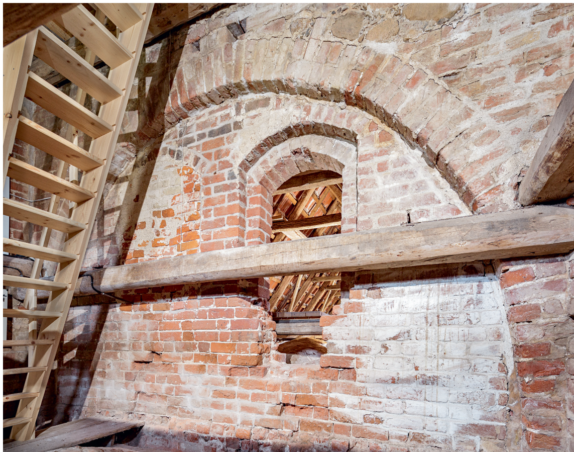
Fig. 9. Mellemstokværkets indre med tårnets oprindelige østgavls inderside med glamhuller (s. 5377 f.) samt aflastningsbue til tårnets forhøjelse (s. 5380). Foto Arnold Mikkelsen 2019. – The interior of the middle floor, showing the inner side of the tower's original east gable with openings, as well as a relieving arch to enable the tower to be of a greater height.
