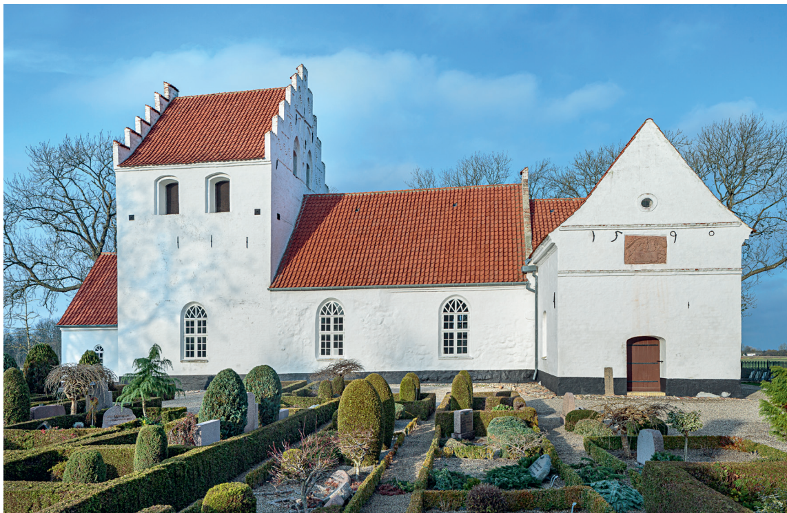
Fig. 7. Kirken set fra syd. Foto Arnold Mikkelsen 2019. – The church seen from the south.
