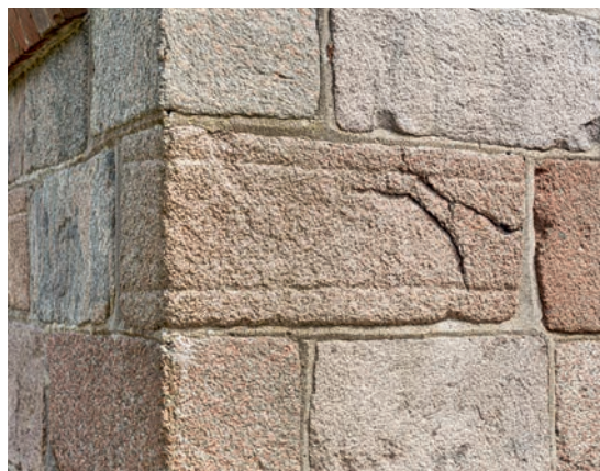
Fig. 8. Kragsten (s. 6002) indmuret i kappellets nordvesthjørne, set fra vest (s. 6016). Foto Arnold Mikkelsen 2020. – Corbelling walled into the north west corner of the chapel, seen from the west.
