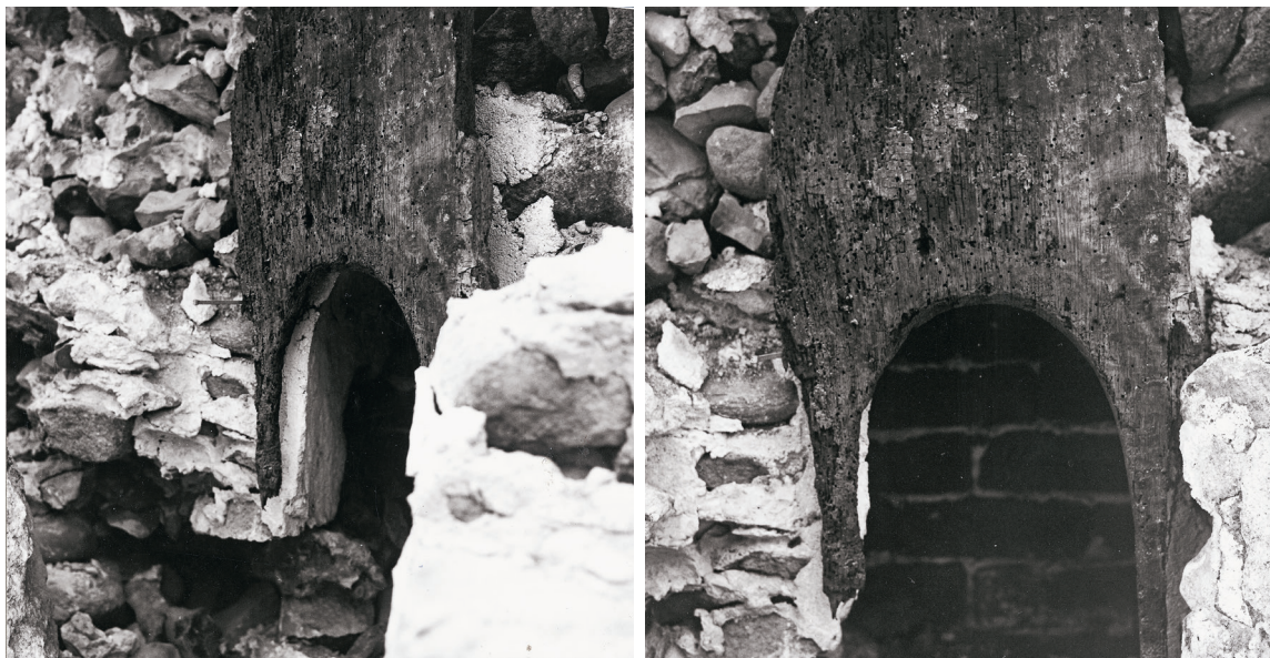
Fig. 104-05. *Romansk vinduesramme under afdækning (s. 6545, jf. s. 6566). 104. Set fra nordvest. 105. Set fra Nord. Foto Birgit Als Hansen 1983. I NM – *Romanesque window frame being uncovered. 104. Seen from the north west. 105. Seen from the north.
