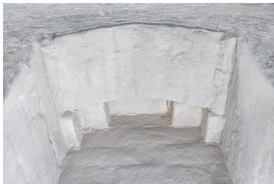
Fig. 18. Fladbuget niche i korforlængelsens sydside (jf. fig. 22, s. 6551), set nedefra. Foto Arnold Mikkelsen 2021. – Segmentally arched niche in the chancel extension's south side (cf. 22), seen from below.
