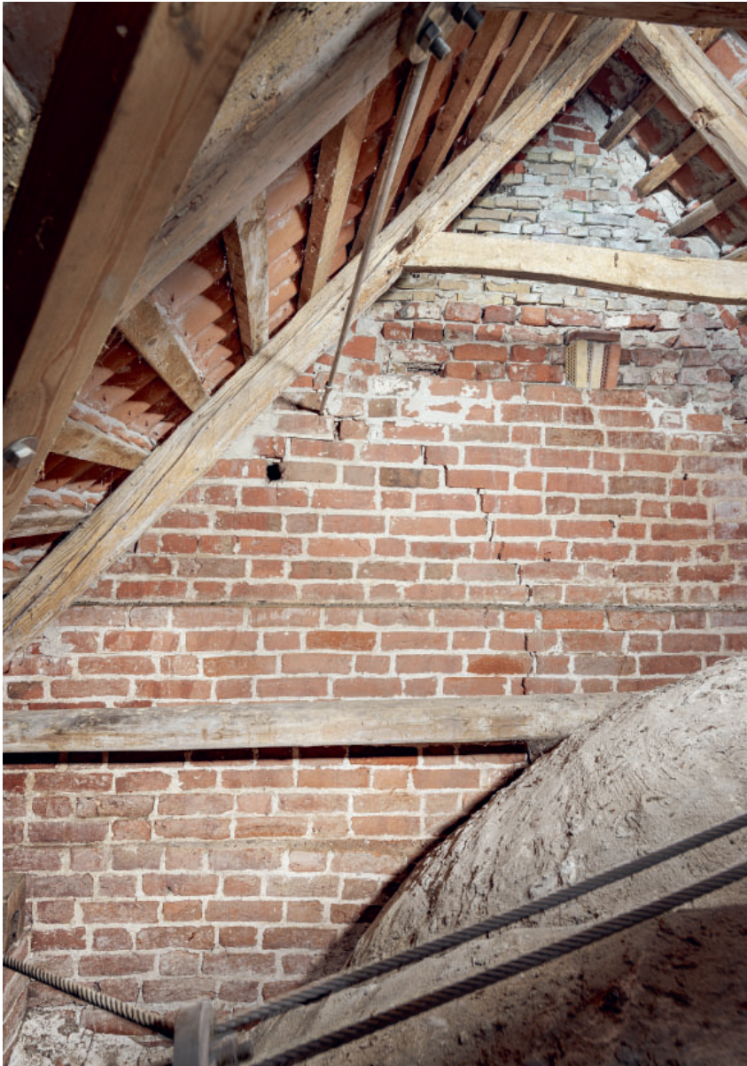
Fig. 24. Korets gavl, fornyet i tegl og med glattede fuger med ridse (s. 6649). Revne i gavlen og fornyet gavltop (s. 6657). Foto Arnold Mikkelsen 2024. – Chancel gable renewed with bricks, and with flush joints and a groove. Crack in the gable and renewed gable top.
