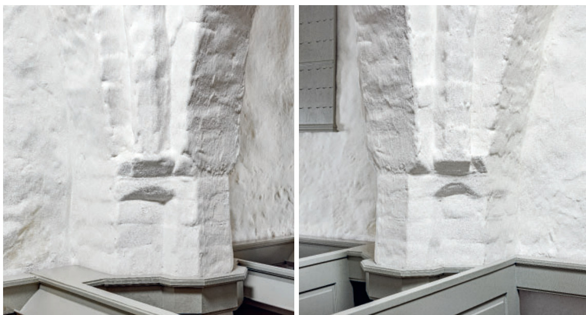
Fig. 10-11. Hvælvpille mellem skibets to fag, i nordsiden (s. 6651). 10. Set mod nordøst. 11. Set mod nordvest. Foto Arnold Mikkelsen 2023. – Vault pier between the two bays of the nave, in the north side. 10. Looking north east. 11. Looking north west.
