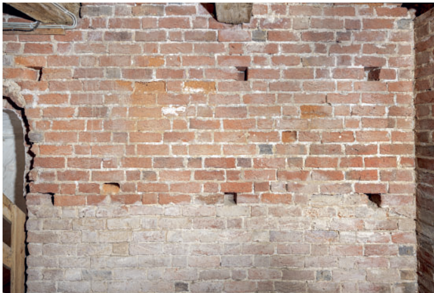
Fig. 32. Tårnets mellemstokværks indre. Sydmur med skalmuring (s. 6747) samt overdørens vestre vange (s. 6748). Foto Arnold Mikkelsen 2023. – Interior of the intermediate floor of the tower. South wall with brick facing, and the western door jamb of the upper door.
