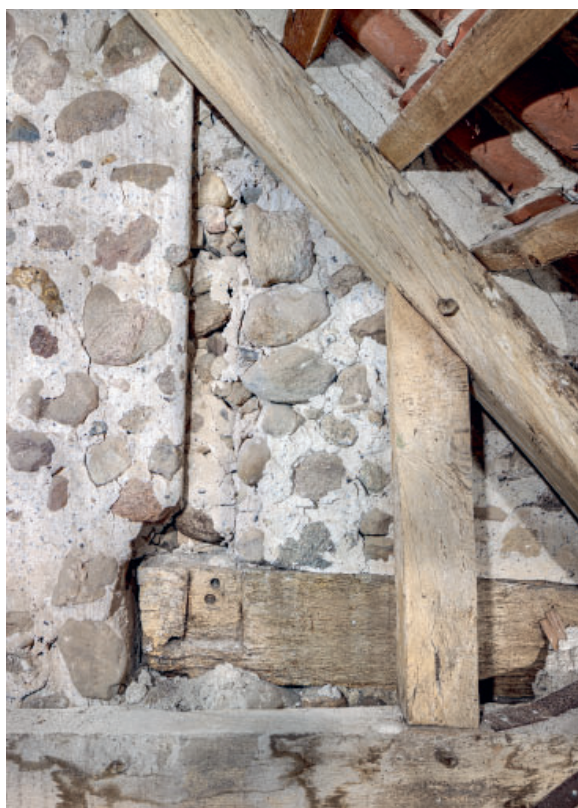
Fig. 39–40. 39. Spor af lodret spærstiver og spærsko i triumfgavlens østside i syd (s. 6862). 40. Spor af lodret spærstiver samt bevaret spærsko i triumfgavlens østside i nord (s. 6862). Foto Arnold Mikkelsen 2024. – 39. Trace of a vertical strut and strutting beam on the east side of the chancel arch gable to the south. 40. Trace of a vertical strut and preserved strutting beam on the east side of the chancel arch gable to the north.
