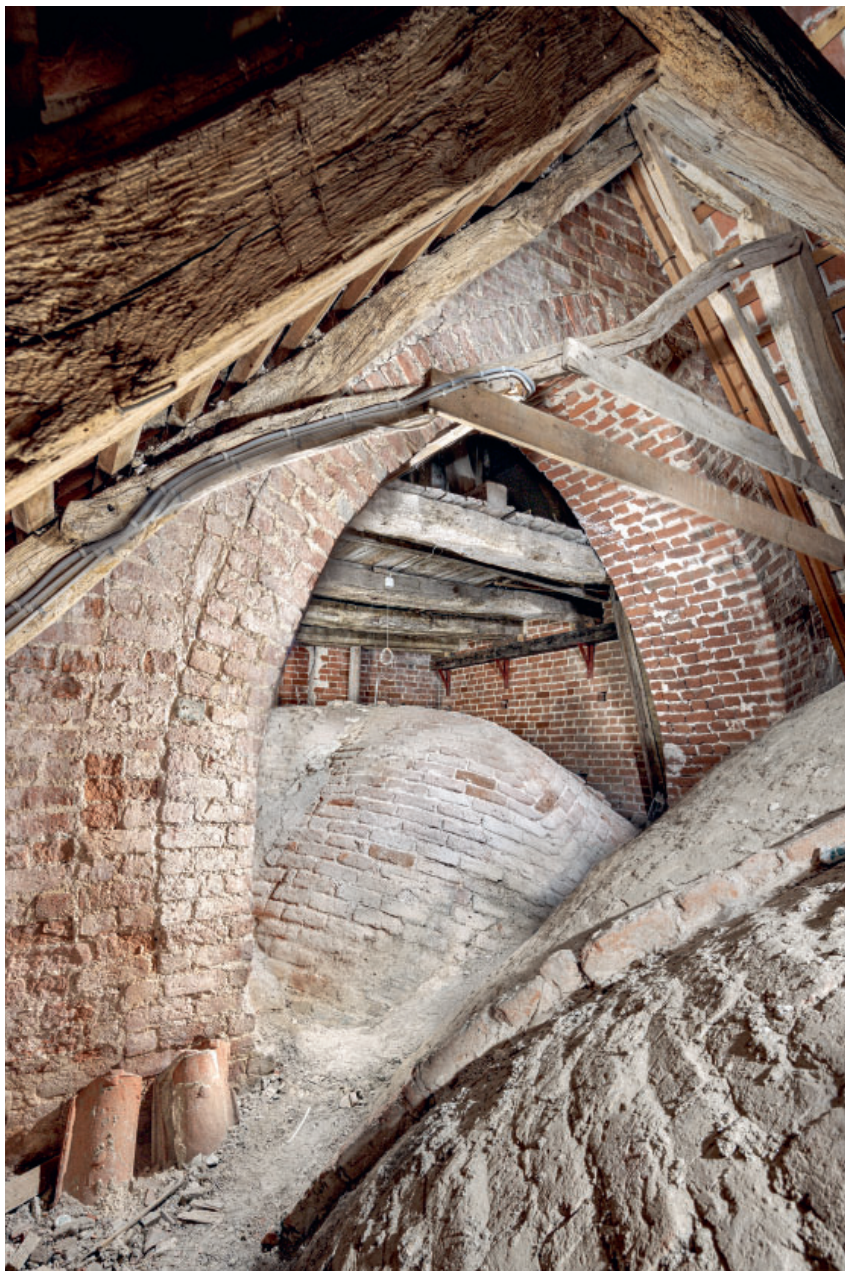
Fig. 29. Aflastningsbue, der bærer tårnets østmur, set mod nordvest (s. 6847). Foto Arnold Mikkelsen 2024. – Relieving arch bearing the east wall of the tower, seen from the north west.
