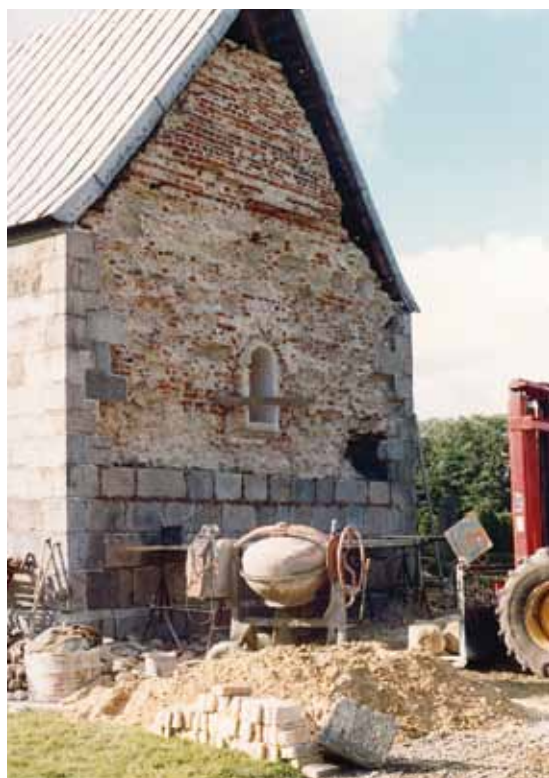
Fig. 59. Korets gavl set fra sydøst under omsætning 1978 (s. 2367). Foto i Struer Museum. – Gable of chancel seen from the south east during resetting.
