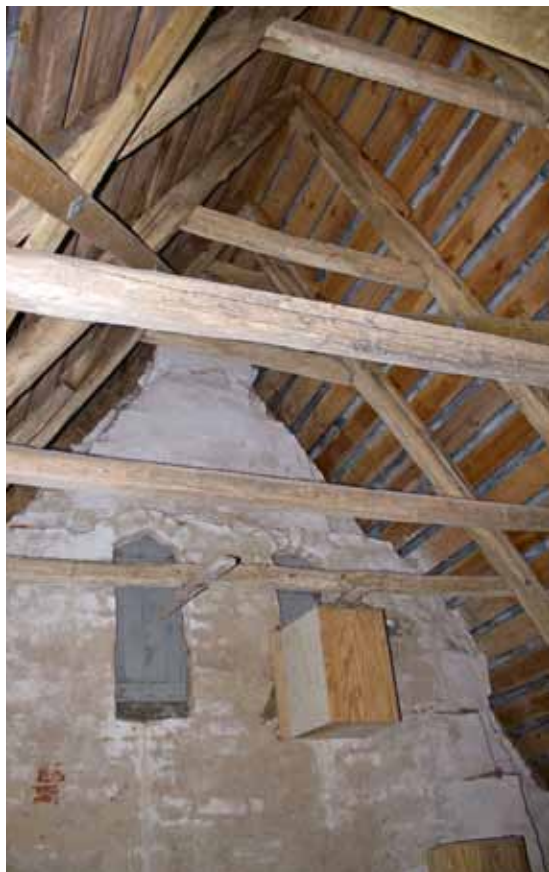
Fig. 49. Tårnets nordre gavltrekant set fra loftet (s. 2409). Foto Anders C. Christensen 2015. – Northern pediment of tower seen from the ceiling.
