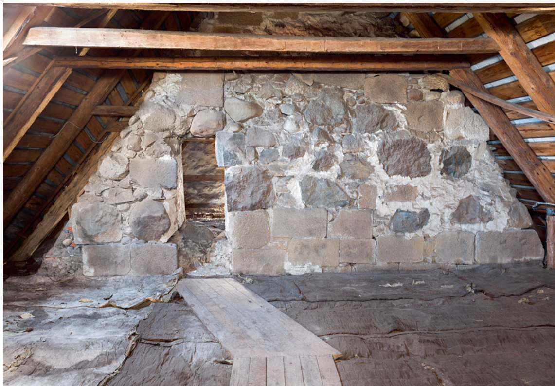
Fig. 13. Skibets loft set mod østre taggavl (s. 2483). Foto Arnold Mikkelsen 2016. – Loft of nave looking towards eastern roof gable.
