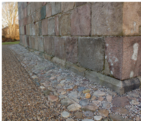
Fig. 12. Sokkel under skibets vestgavl set fra sydvest (s. 2481). Foto Anders C. Christensen 2017. – Footing beneath west gable of nave seen from the south west.
