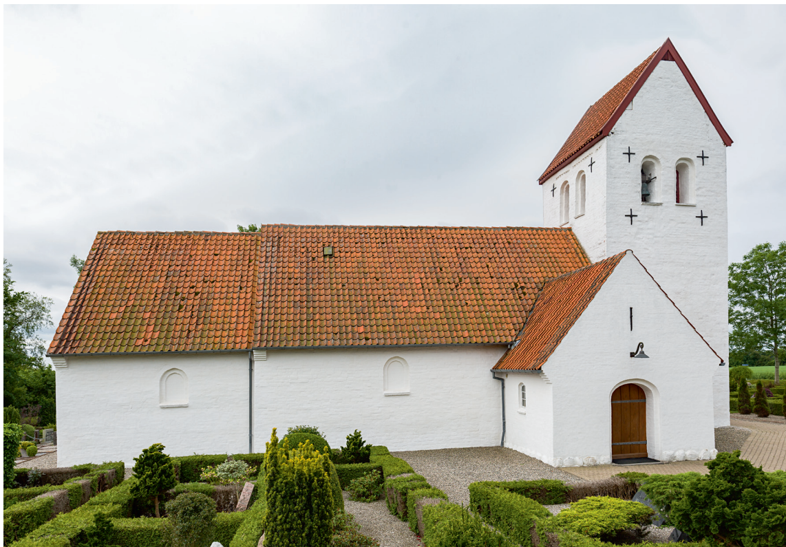
Fig. 6. Ydre set fra nord. Foto Arnold Mikkelsen 2017. – Exterior seen from the north.
