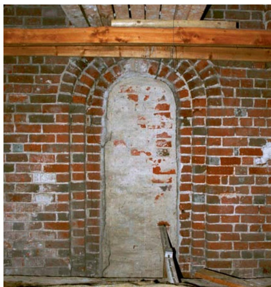
Fig. 51. Korforlængelsens nordvindue set fra sakristiets loftsrums. Foto Mogens Vedsø 2011. – The north window of the chancel extension seen from the loft of the vestry.
