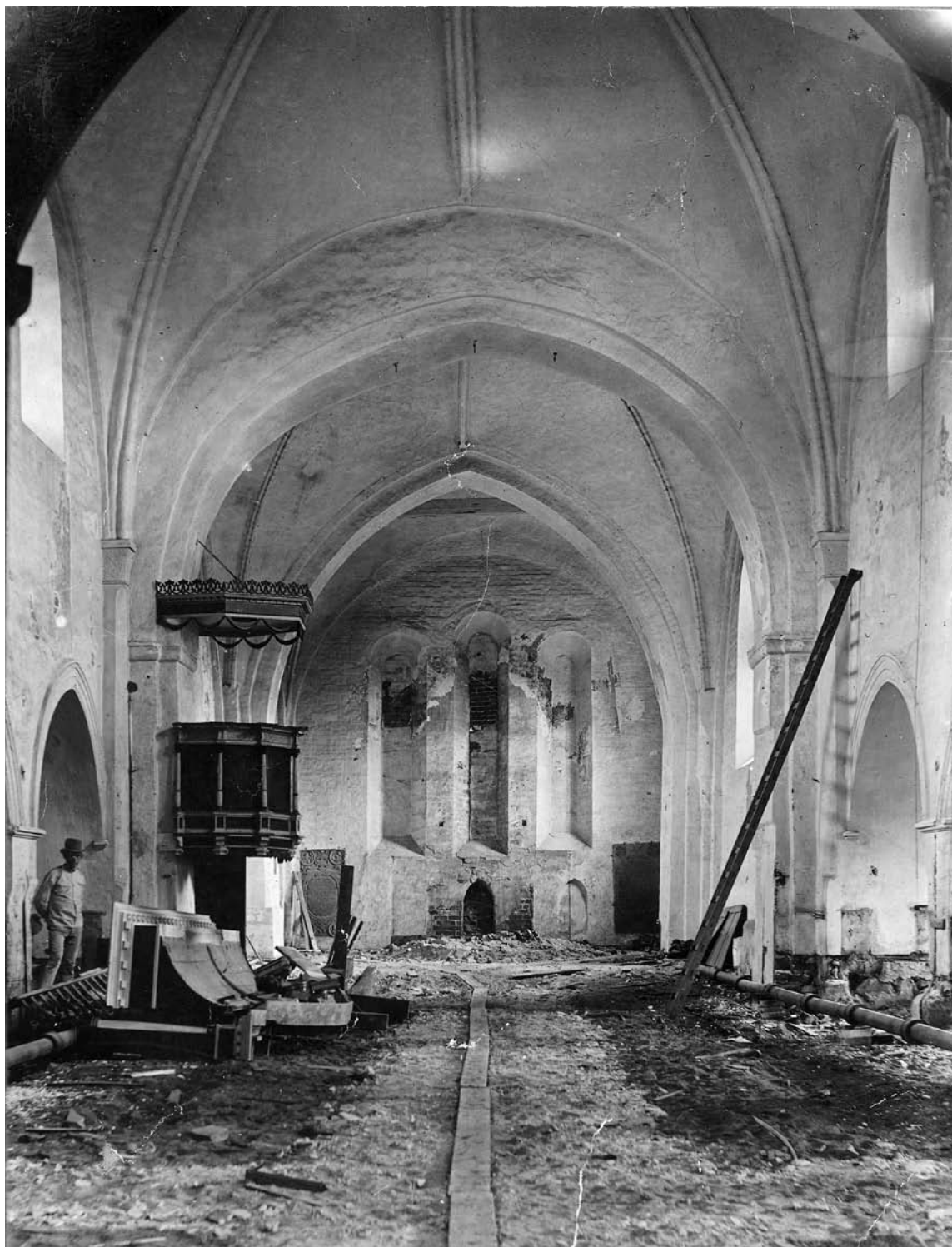
Fig. 48. Kirkens indre set mod øst under Storcks restaurering 1892. Under det trekoblede vindue ses de to bevarrede nicher (s. 142). Foto 1892. — Interior of the church, looking east, during Storck's restoration in 1892. Under the triforium window the two preserved niches can be seen.
