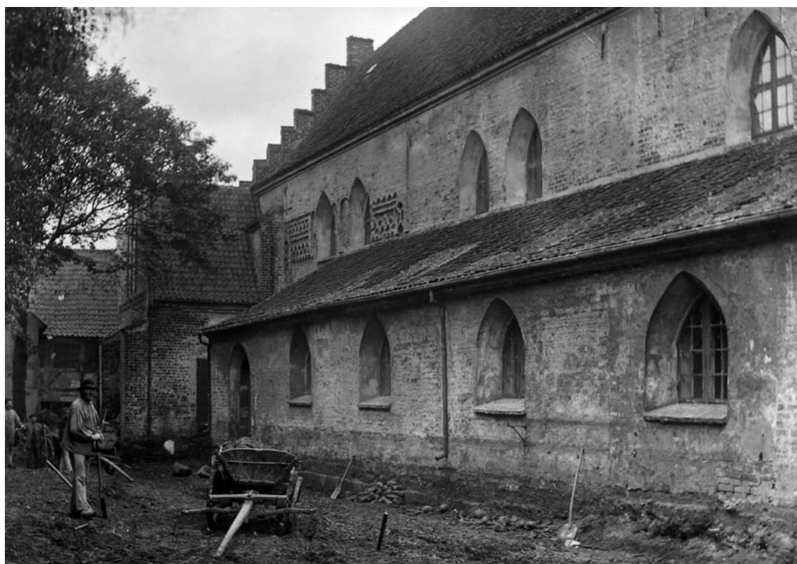
Fig. 42. Nordre sideskib set fra nordvest under H. B. Storcks restaurering. Foto Johan Hermann 1892. – North side-aisle seen from northwest during H. B. Storck's restoration.
