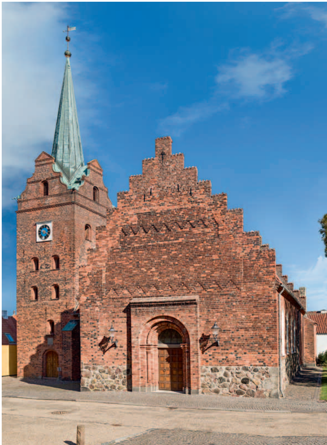
Fig. 26. Kirken set fra sydvest. Foto Arnold Mikkelsen 2015. – The church seen from the south west.
