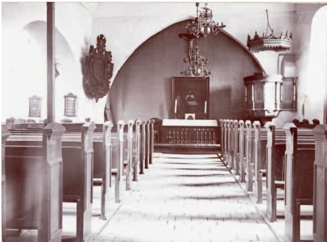
Fig. 42. Indre set mod øst under restaureringen o. 1895. †Hvælvene i koret er nedtaget. I den gamle †korbue, der kort efter blev nymuret, ses bag prædikestolen rester af skibets gamle østvæg (s. 1379). Foto i Rudkøbing Byhistoriske Arkiv. – Interior looking east during the restoration c. 1895. †The vaults in the chancel have been taken down. In the old †chancel arch, which was rebuilt shortly afterwards, remains of the old east wall of the nave can be seen behind the pulpit.
