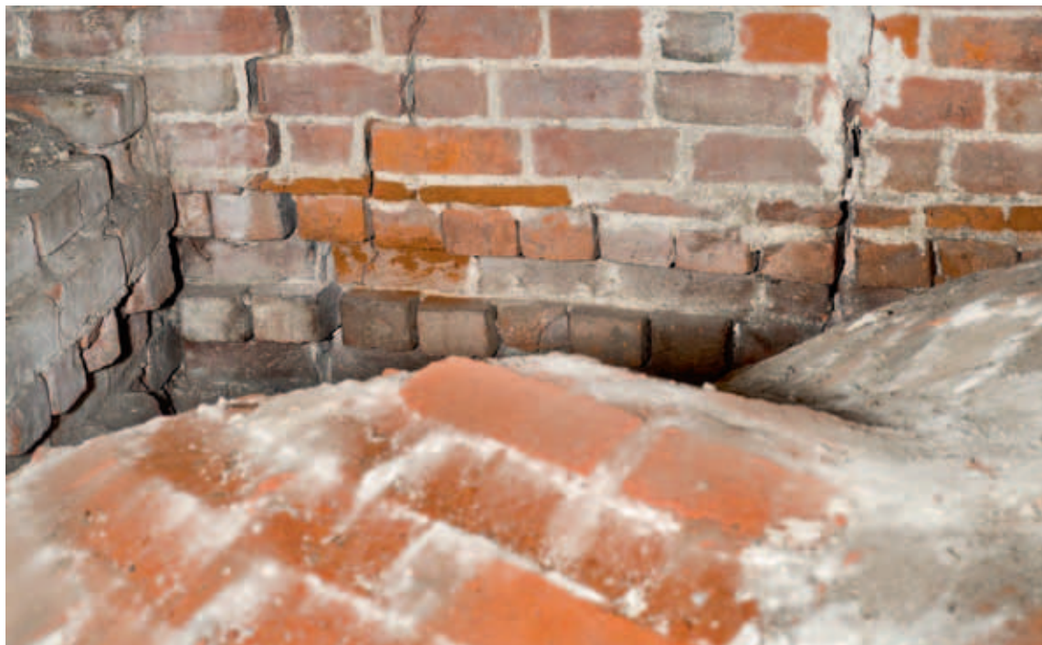
Fig. 24. Hvælvfortandinger set fra sakristiets loft, øverst i korets nordmur og i sakristiets østvæg (tv.) (s. 1379). Foto Arnold Mikkelsen 2015. – Vault toothings seen from the ceiling of the sacristy, at the top of the north wall of the chancel and in the east wall (left) of the sacristy.
