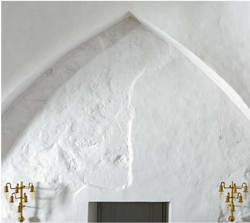
Fig. 8. Tilmuret romansk vindue i korets nordmur (s. 2069). Foto Arnold Mikkelsen 2018. – Bricked-up Romanesque window in north wall of chancel.
