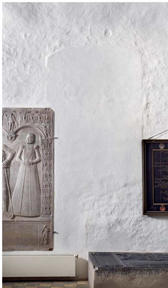
Fig. 33. Kurvehanksformet \dagger vindue i søndre korsarms østmur (s. 2237). Foto Arnold Mikkelsen 2019. – Basket-handle \dagger window arch in the east wall of the south transept.
