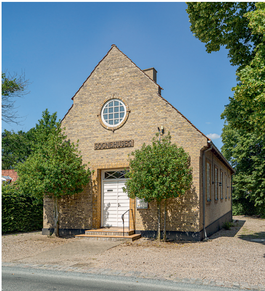
Fig. 1. Kirkesalen set fra sydvest. Foto Arnold Mikkelsen 2020. – Church hall seen from the south west.
