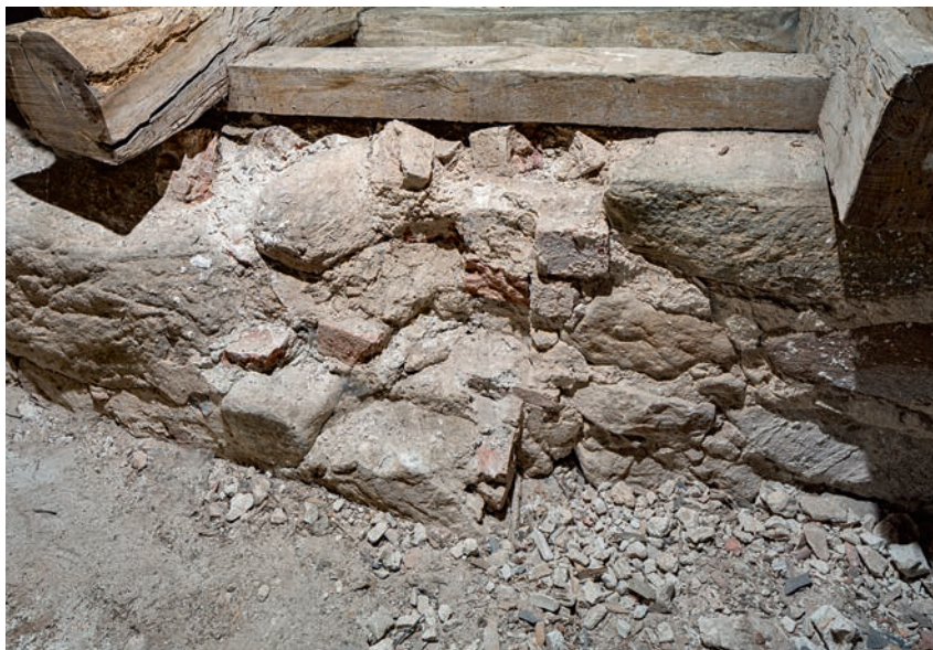
Fig. 11. Lodfuge i langhusets sydside (s. 2941). Foto Arnold Mikkelsen 2019. – Soldered joint in the south side of the nave.
