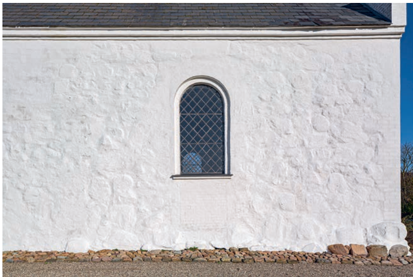
Fig. 98. Korets sydfacade (s. 2944). Foto Arnold Mikkelsen 2019. – South facade of the chancel.
