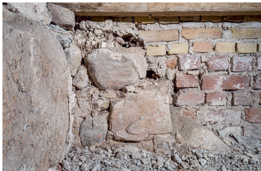
Fig. 68. Rest af skibets nordmur set fra nordkappellets loft (s. 3027). Foto Arnold Mikkelsen 2019. – Remains of north wall of nave seen from loft of north chapel.
