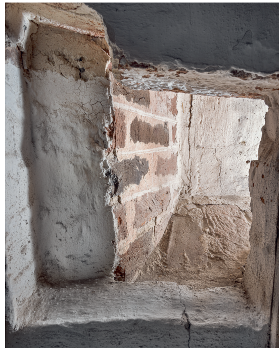
Fig. 173. Smiget vinduesvange med rester af rød kalk og hvide, opmalede fuger. Tilmuret vindue i søndre høj Kirkemurs andet fag set mod nord (s. 3356). Foto Arnold Mikkelsen 2021. – Bevelled window side member with traces of red lime wash and white, painted-up joints. Bricked-up window in the second bay of the southern high church wall, looking north.
