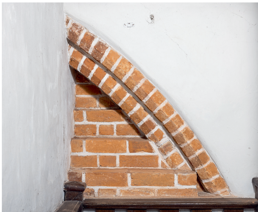
Fig. 40. Detalje af den østligste sideskibsarkade i kirkens sydmur set mod nord (s. 3350). Foto Arnold Mikkelsen 2021. – Detail of the easternmost side-aisle arcade in the south wall of the church, looking north.
