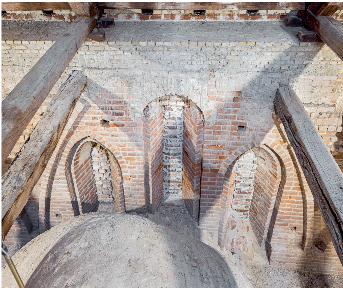
Fig. 50. Søndre højkirkemurs 4. vinduesfag set mod syd (s. 3357). Foto Arnold Mikkelsen 2021. — The fourth window bay of the southern high church wall, looking south.
