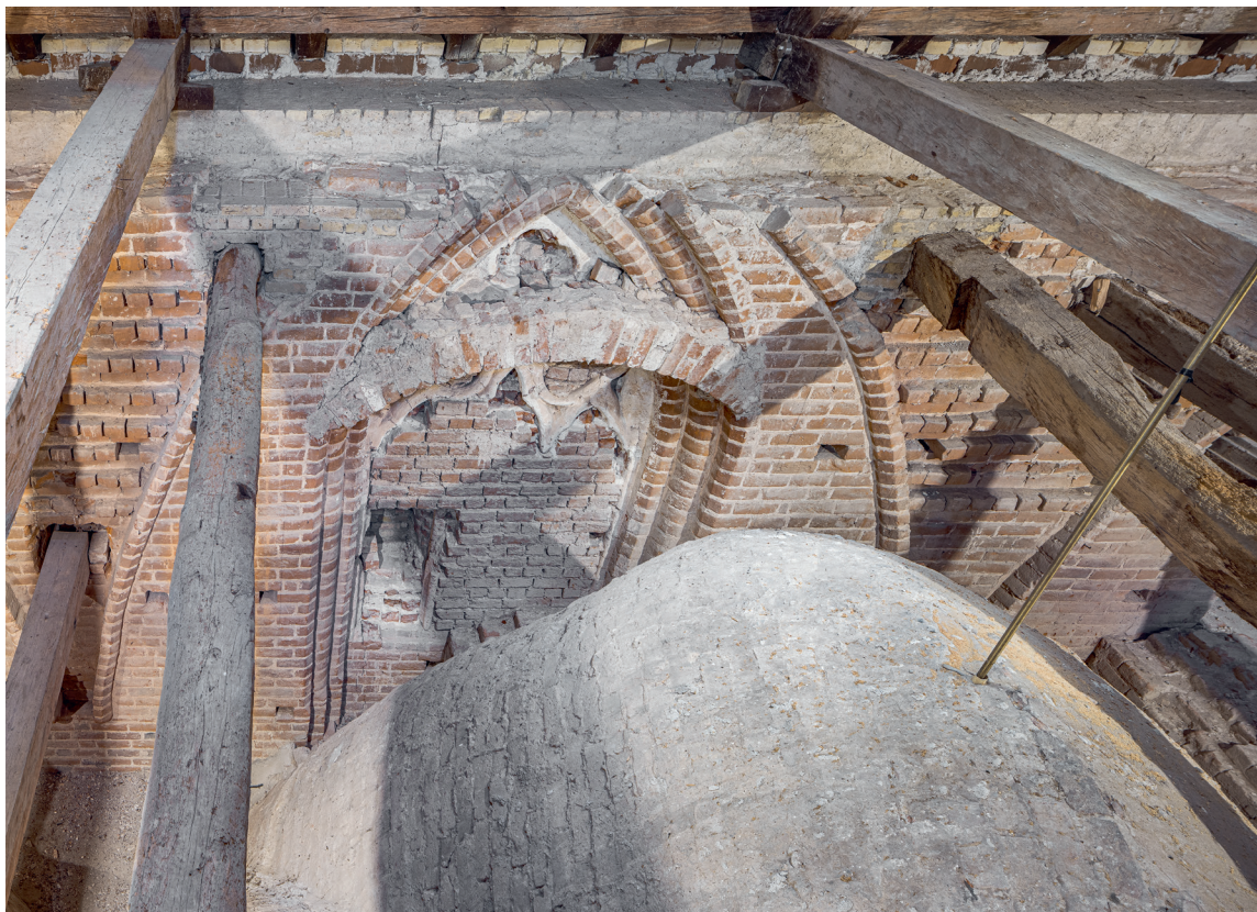
Fig. 64. Nordre højkirkemurs fjerde vinduesfag set mod nord (s. 3365). Foto Arnold Mikkelsen 2021. – The fourth window bay of the northern high church wall, looking north.
