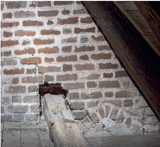
Fig. 172. Søndre høj Kirkemur set fra østfløjens loft. Bemærk resterne af facadens røde kalk med hvide, opmalede fuger (s. 3356). Foto Arnold Mikkelsen 2021. – Southern high church wall seen from the loft of the east wing. Note the traces of the facade's red lime wash with white, painted-up joints.
