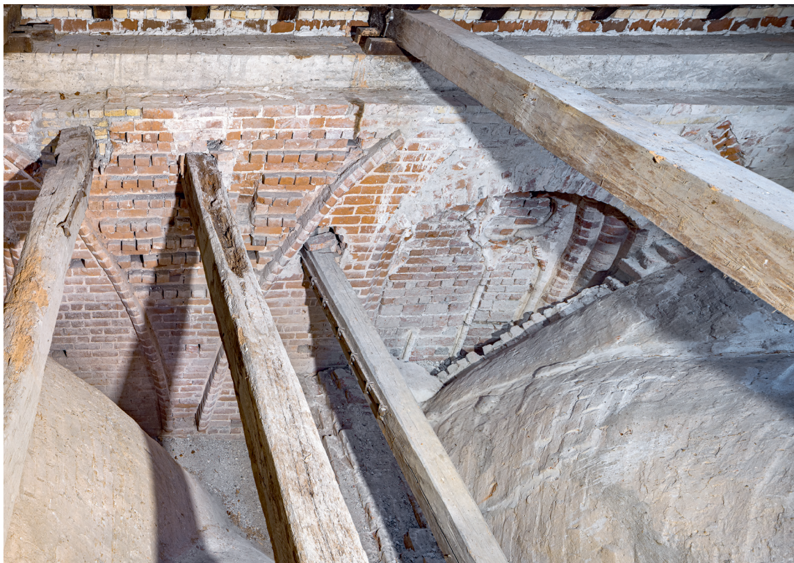
Fig. 62. Nordre høj Kirkemurs 3. vinduesfag og hvælvfortanding mellem 3. og 4. fag set mod nord (s. 3365–67). Foto Arnold Mikkelsen 2021. — The third window bay and vault toothing of the northern high church wall between the third and fourth bay, looking north.
