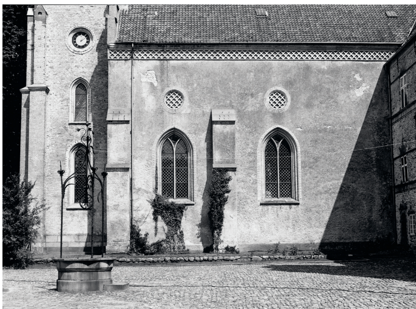
Fig. 84. Kirkens sydfacade set fra syd. Foto Jens Chr. Varming 1988-89. I Varmings Tegnesteue. — The south facade of the church seen from the south.
