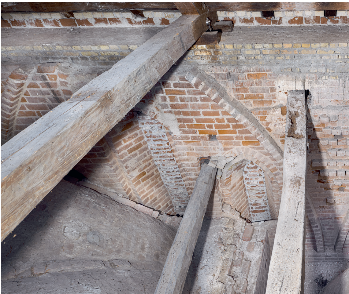
Fig. 49. Søndre højkirkemurs 3. vinduesfag og hvælvfortanding mellem 3. og 4. fag set mod syd (s. 3357). Foto Arnold Mikkelsen 2021. – The third window bay of the southern high church wall and vault toothing between the third and fourth bay, looking south.
