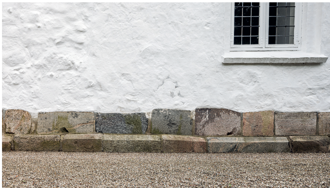
Fig. 9. Romanske sokkelsten i kirkens nordmur (s. 3689). Foto Arnold Mikkelsen 2022. – Romanesque footing stones in the north wall of the church.
