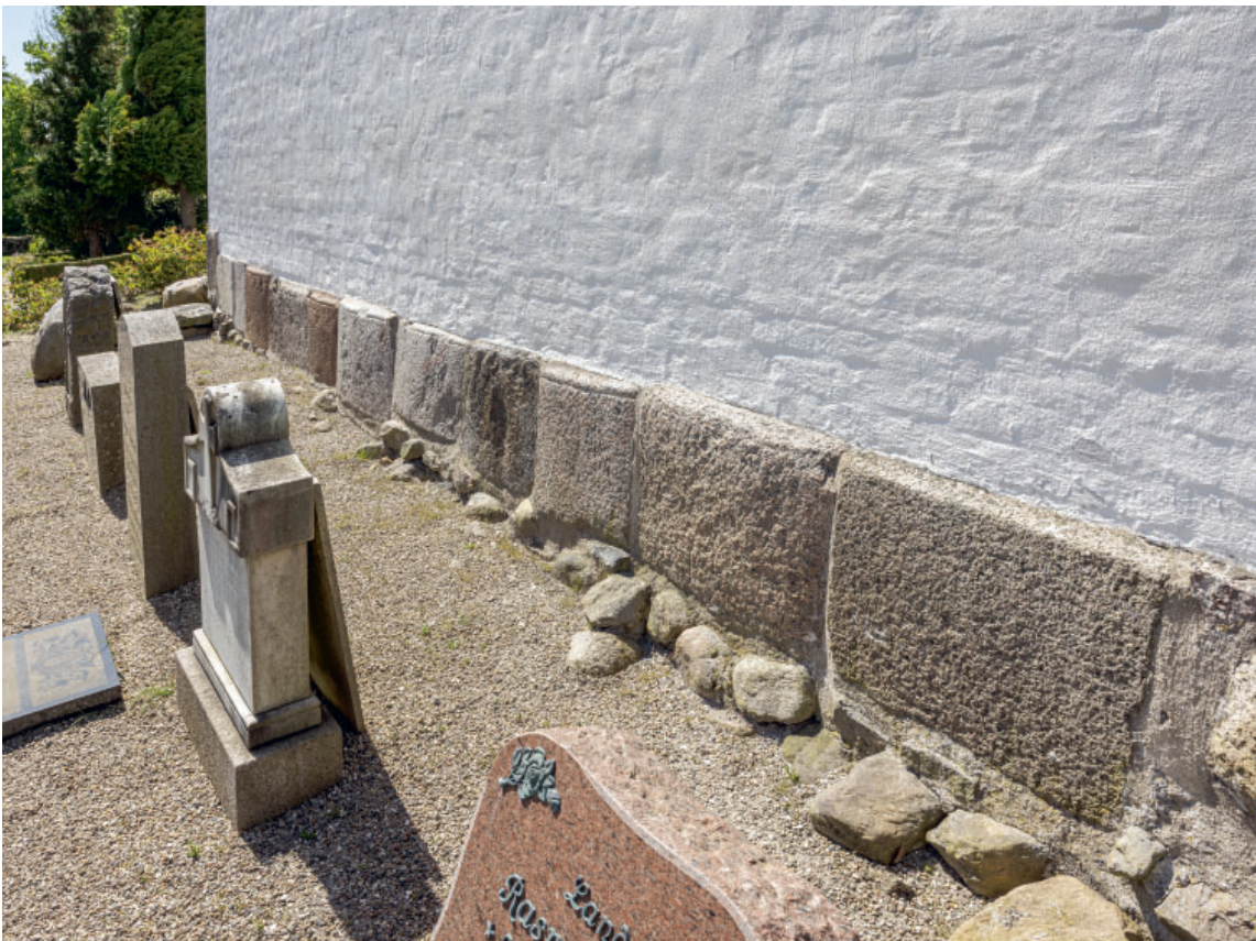
Fig. 11. Sokkelsten fra romansk \dagger apsis i langhusets østgavl (s. 4286). Foto Arnold Mikkelsen 2024. – Footing stones from the Romanesque \dagger apse in the nave-chancel's east gable wall.
