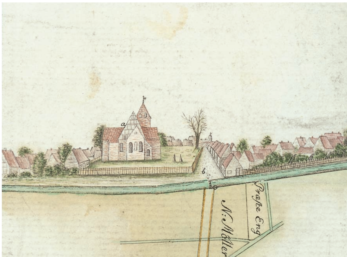
Fig. 2. Kirken og kirkegården set fra det ubeboede terræn øst for Mølleåen 1802. Kirken ses med sit oprindelige \dagger kor og \dagger sakristiet (s. 104) ved dets nordside, begge nedrevet 1855. Skibets store gavnl er i bindingsværk. På den græsklædte kirkegård ses to monumenter (s. 184). Koloreret tuschtegning ved S. Ravn i RA. – The church and churchyard viewed from the uninhabited terrain east of Mølleåen, 1802. The church is seen with its original \dagger chancel and \dagger sacristy on its north side, both demolished in 1855. The large gable of the nave is in half-timbering. In the grassy churchyard we see two monuments.
