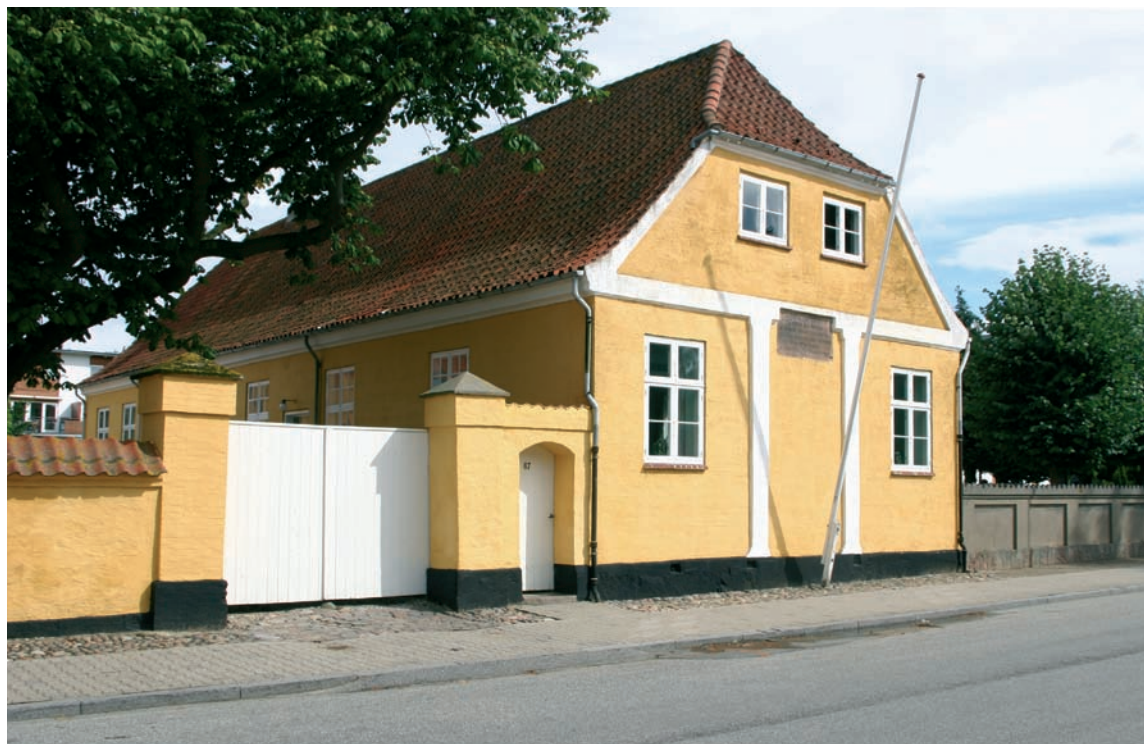
Fig. 5. Den tidligere skoles vestgavl mod Dronningensgade (s. 502). Foto Hugo Johannsen 2006. — The west gable of the former school towards Dronningensgade.
