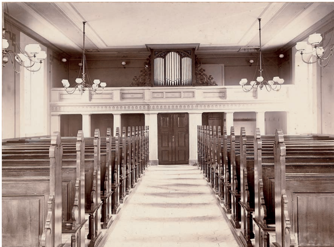
Fig. 18. Indre set mod nord. Foto 1901 ved embedet. – Interior viewed towards the north.
