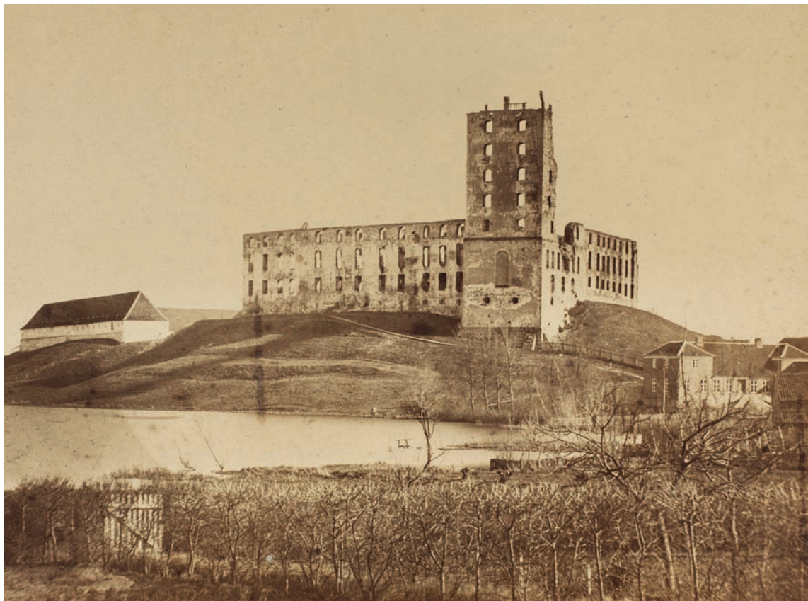
Fig. 1. Slotsruinen set fra nord. Ældre foto i KglBibl. – The castle ruin seen from the north.
