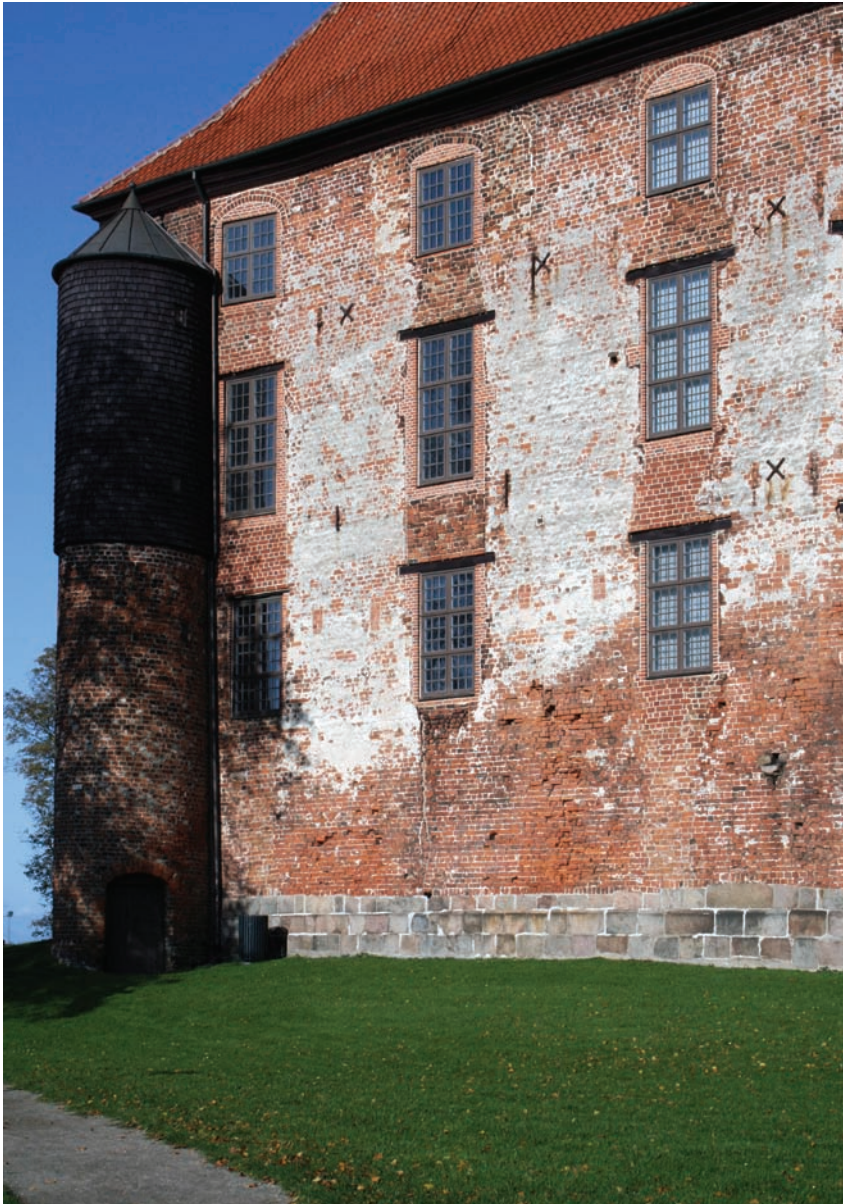
Fig. 10. Sydfacade af Christian III's (†)slotskirke (s. 936). Foto Hugo Johannsen 2008. – South facade of Christian III's (†)Castle Chapel.
