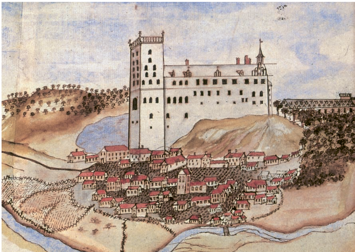
Fig. 5. Koldinghus set fra vest efter Christian IV's ombygning 1598-1616. Udsnit af tegning o. 1660, tilskrevet prins Christian (V). Rosenberg, – Koldinghus seen from the west after Christian IV's rebuilding in 1598-1616. Section of drawing from c.1660, attributed to Prince Christian (V).
