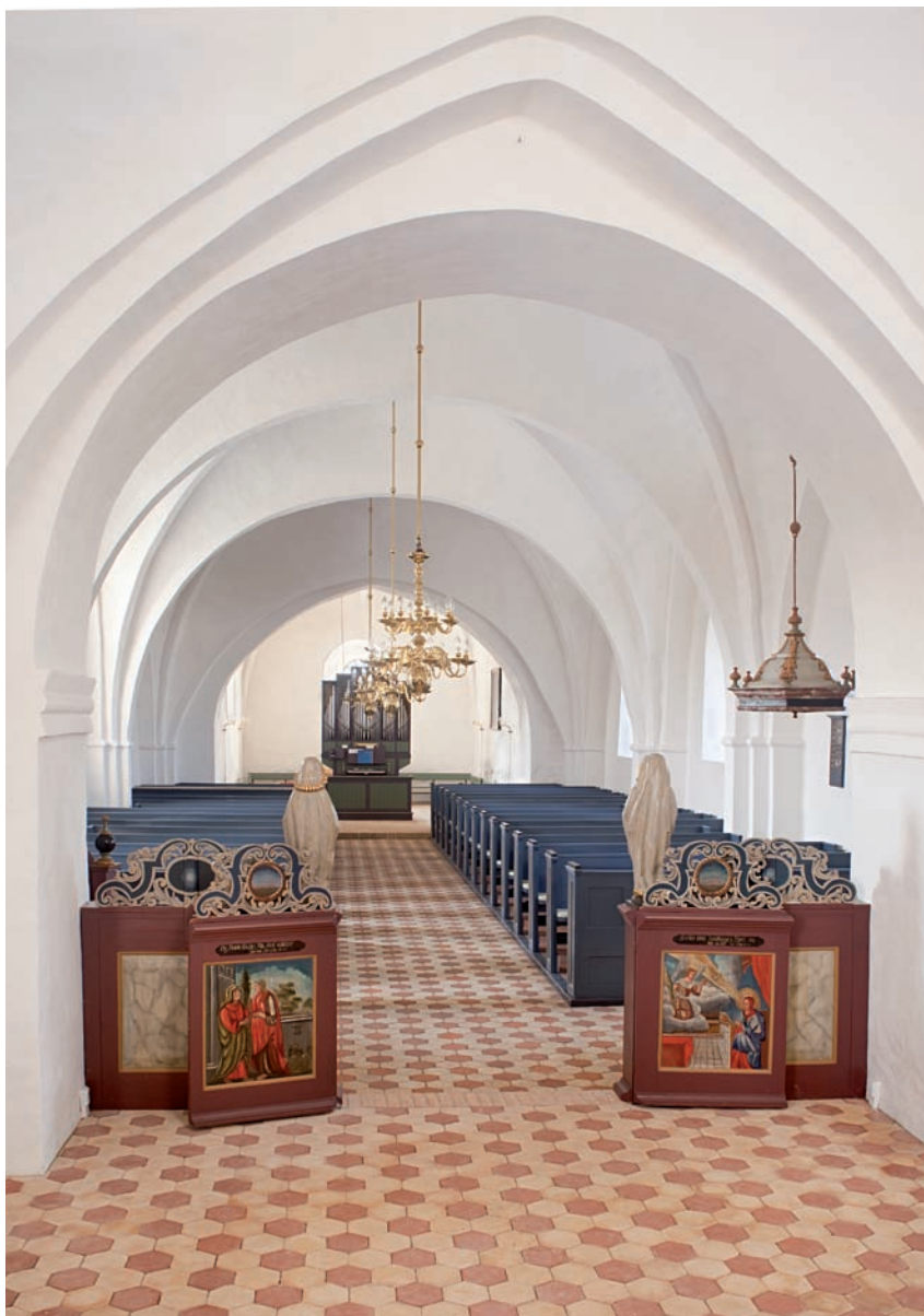
Fig. 37. Indre set mod vest. Foto AM 2009. – Interior looking west.
