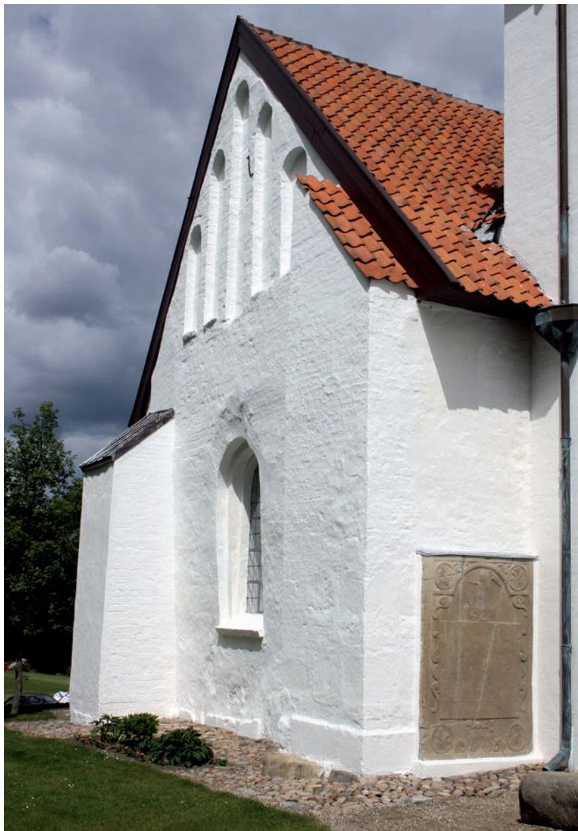
Fig. 8. Skibets vestgavl set fra sydvest. Foto EN 2009. – The west gable of the nave, seen from the southwest.
