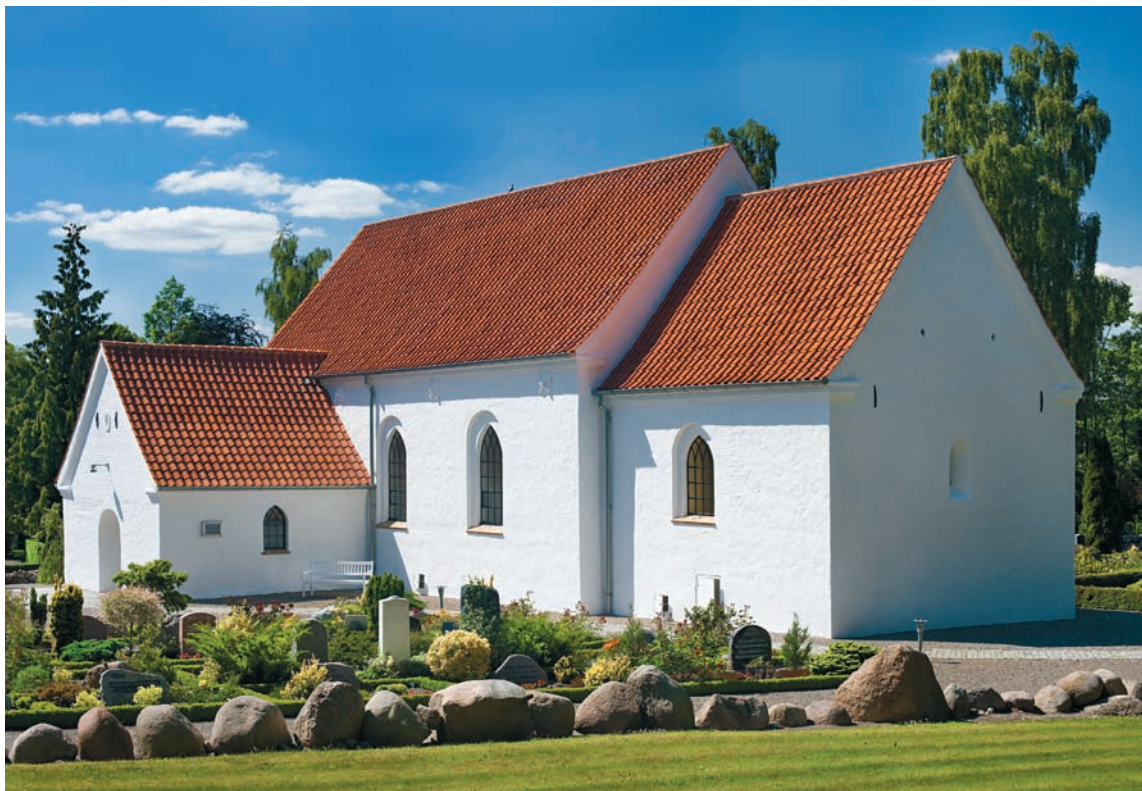
Fig. 1. Kirken set fra sydøst. Foto AM 2009. – The church seen from the southeast.
