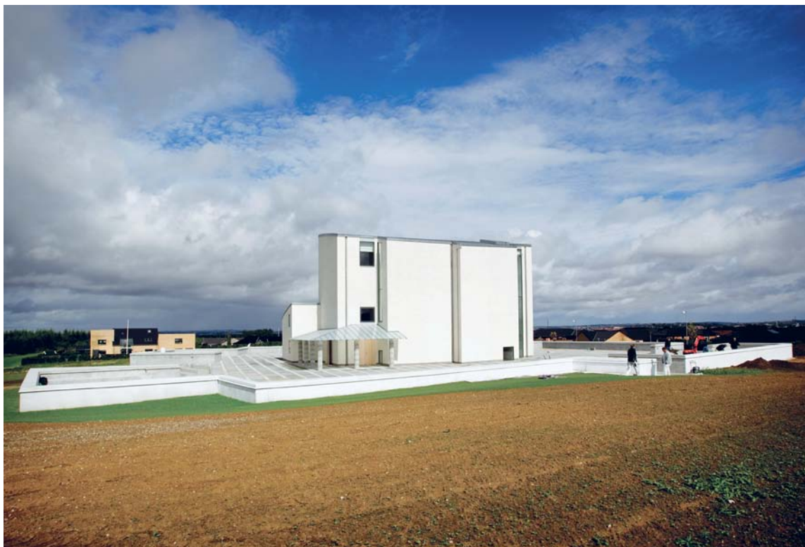
Fig. 3. Kirken og kirkepladsen set fra syd under opførelsen 2011. Foto Morten Pape. – Church and church square seen from the south during construction, 2011.
