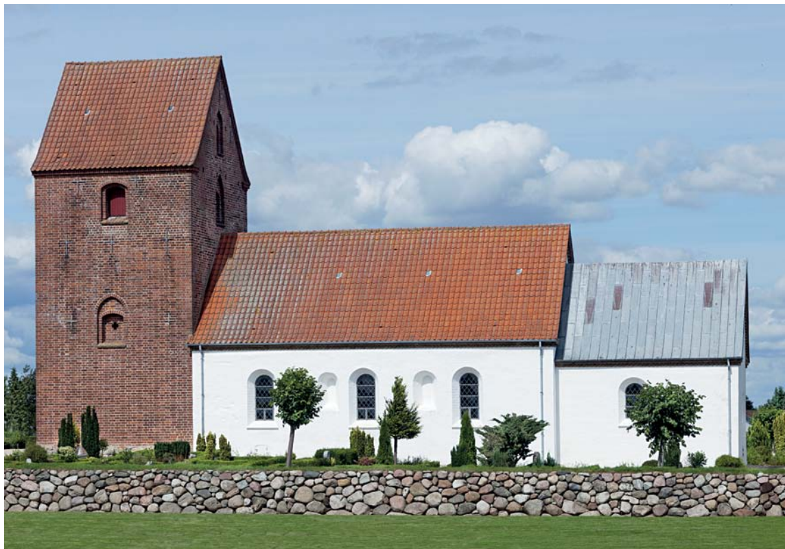
Fig. 1. Kirken set fra syd. Foto AM 2012. – The church seen from the south.
