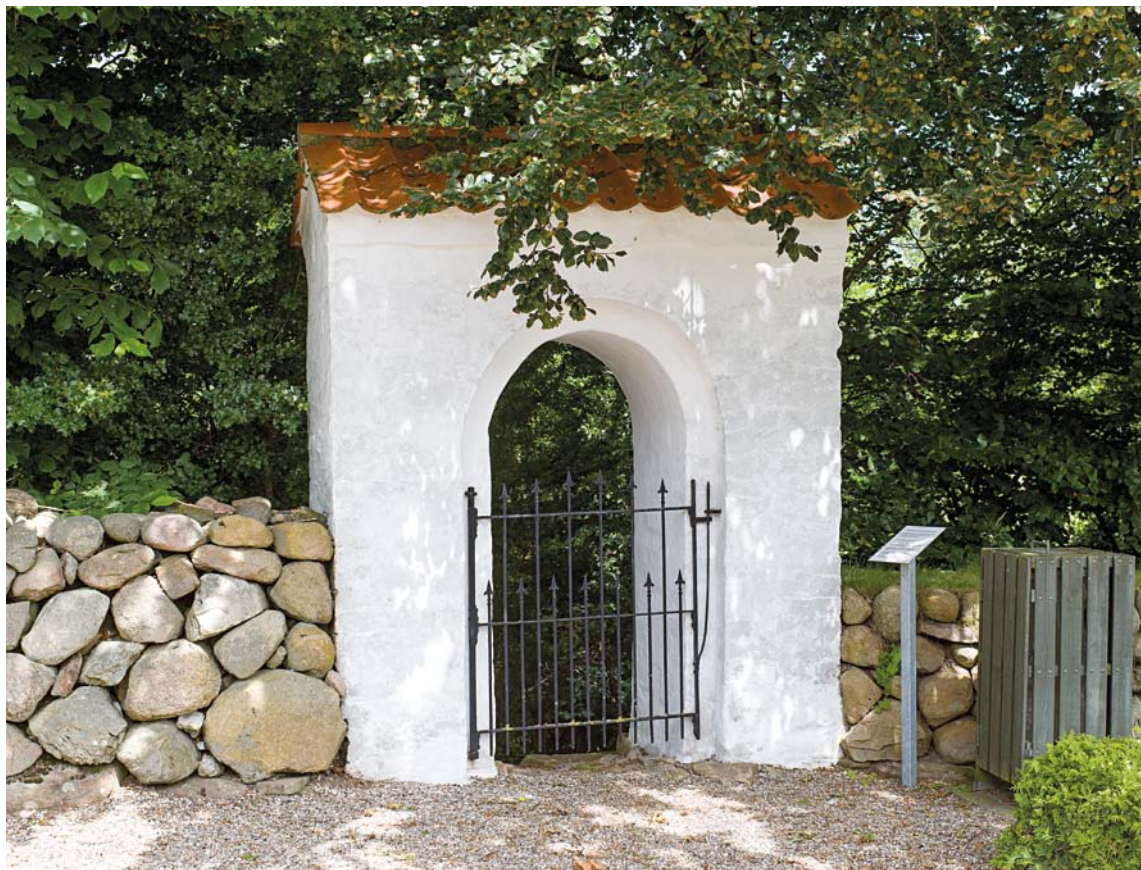
Fig. 4. Kirkegårdsportal i norddiget, senmiddelalderlig, set fra syd (s. 1993). Foto Arnold Mikkelsen 2014. – Churchyard gate in the north wall, Late Medieval, seen from the south.
