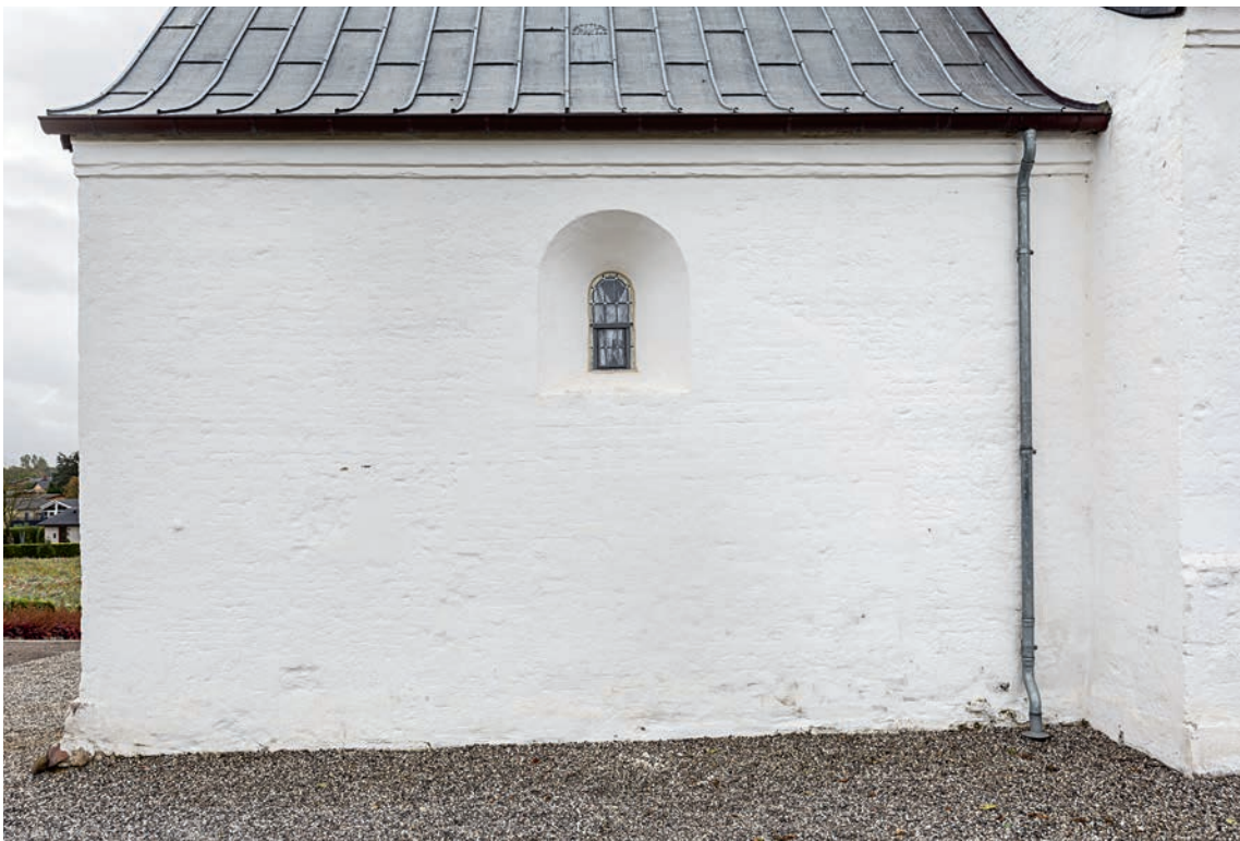
Fig. 10. Koret set fra nord. Foto Arnold Mikkelsen 2016. – The chancel seen from the north.
