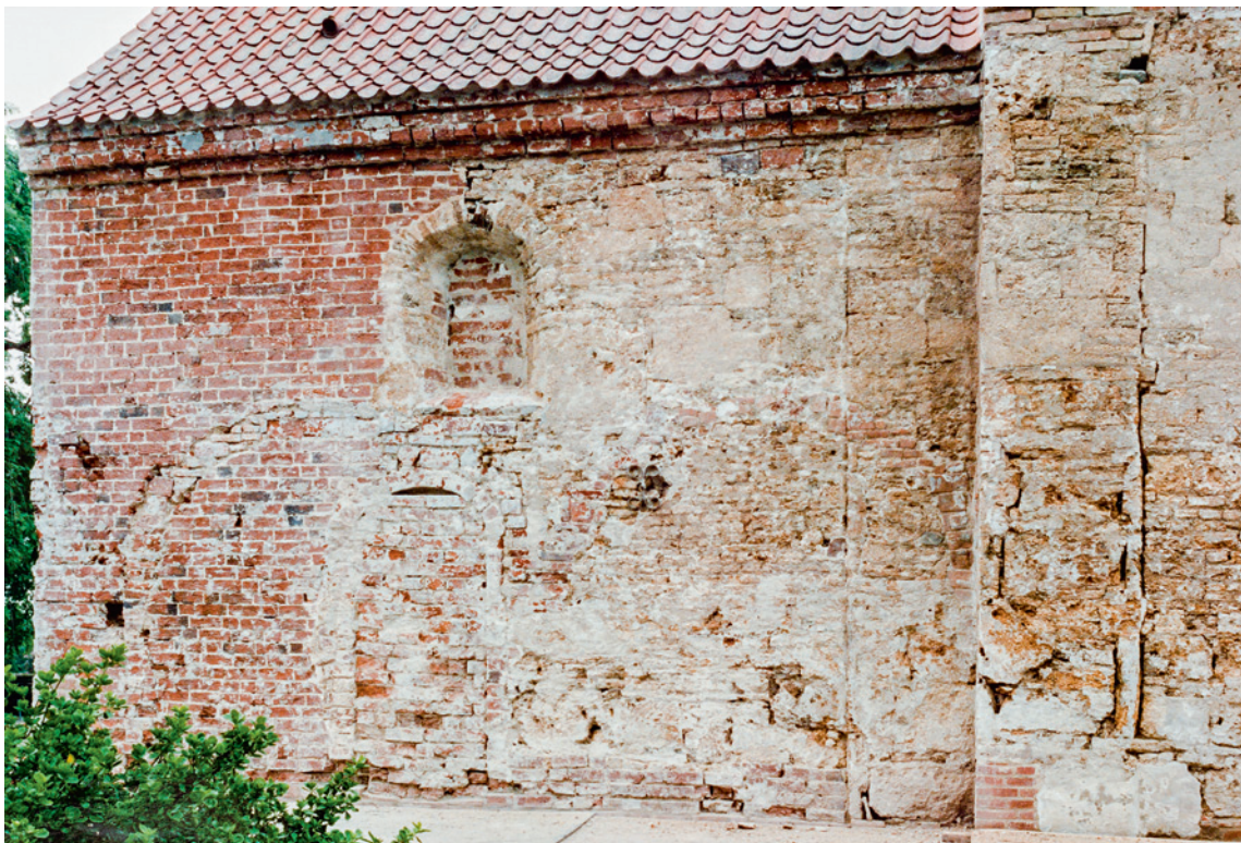
Fig. 13. Korets nordmur under restaureringen 1989-92. Give-Egnens Museum. – North wall of the chancel during restoration 1989-92.
