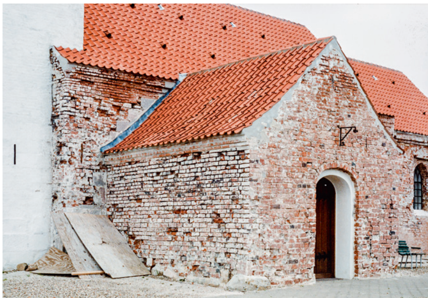
Fig. 20. Våbenhuset under restaureringen 1989-92 set fra sydvest. Give-Egnens Museum. – The porch during restoration 1989-92 seen from the south west.
