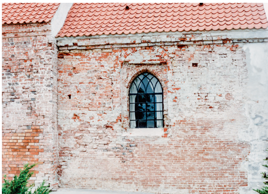
Fig. 16. Korets sydmur under restaureringen 1989-92. Give-Egnens Museum. — South wall of the chancel during restoration 1989-92.
