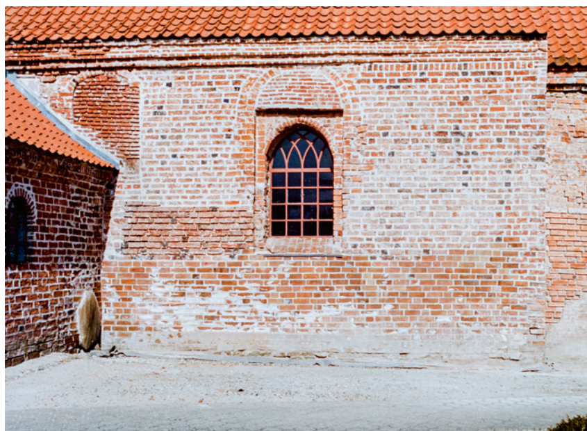
Fig. 14. Udsnit af skibets sydmur under restaureringen 1989-92. Give-Egnens Museum. – South wall of the nave during restoration 1989-92.
