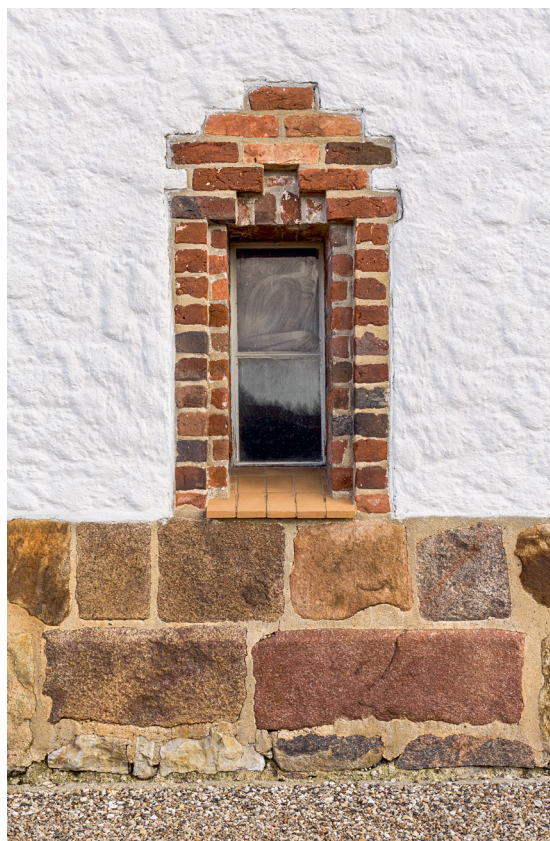
Fig. 39. Tårnets vestvindue sat i sten udgravet i teglovnen (s. 2861). Foto Arnold Mikkelsen 2019. – West window of the tower set with bricks excavated in the brick kiln.
