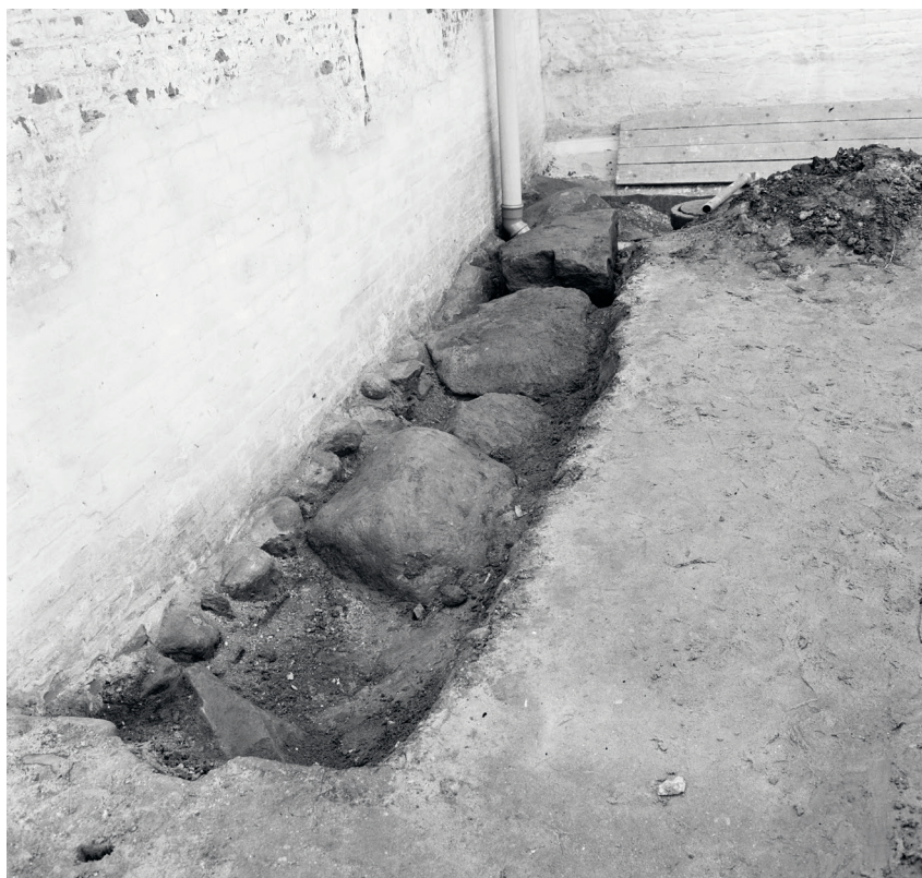
Fig. 147. Frilagt fundament langs våbenhusets østmur set fra syd (s. 3057). Foto Knud J. Krogh 1976. – Exposed foundation along the east wall of the porch seen from the south.
