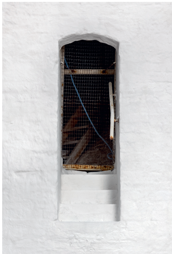
Fig. 66. Tårnets dør i andet stokværk, set fra nord. Foto Inger Marie Helgasmøller Mulvad 2021. – Door of the tower on second storey, seen from the north.
