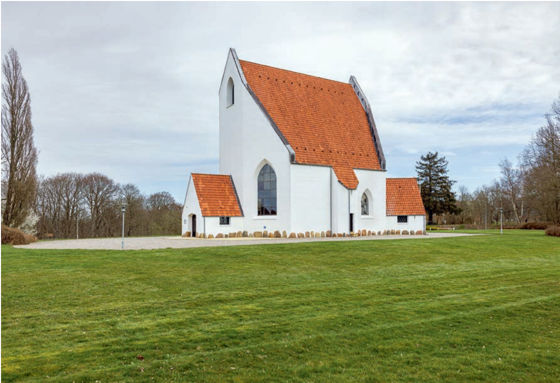
Fig. 1. Ydre set fra sydvest. Foto Arnold Mikkelsen 2023. – The exterior seen from the south-west.
