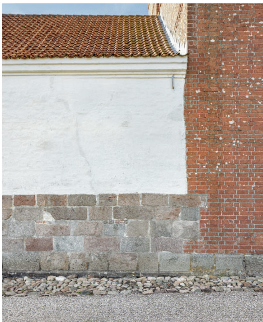
Fig. 14. Overgangen mellem vestforlængelsen og tårnet set fra nord. Foto Arnold Mikkelsen 2023. – The transition between the western extension and the tower seen from the north.
