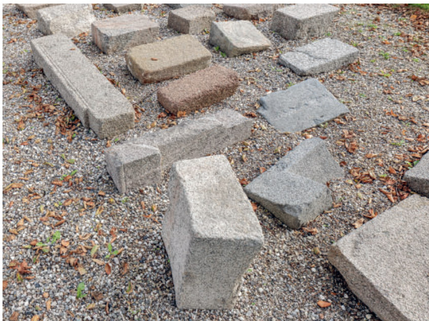
Fig. 9. Udvalg af kvadre opbevaret øst for diget (s. 4161, jf. fig. 80): krumhugget kvader (s. 4167), aflang karmsten med rundstav (s. 4164), samt sålbænksten mv. Foto Arnold Mikkelsen 2023. – Selection of ashlar stored east of the churchyard wall (cf. fig. 80): curved ashlar, oblong casing stone with astragal, as well as sill stone etc.
