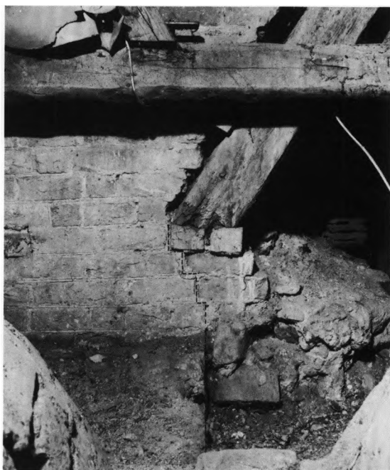
Fig. 12. Langhusets sydmur med sekundær falsgesims af tegl, set fra loftsrummet mod det sekundært tilbyggede tårns østside (s. 1303). Til venstre anes søndre sideskibs vestligste hvælv, hvis nordvestre hvævlomme er muret ud mod den senere nedrevne del af langhusets sydmur (s. 1309, jfr. fig. 4). HJ fot. 1984. - South wall of the long-house with brick cornice, seen from the loft towards the east side of the secondary tower. To the left, the south side aisle's most westerly vault is faintly discernible. The north-west spandrel was originally abutting the south wall before its partial removal.
