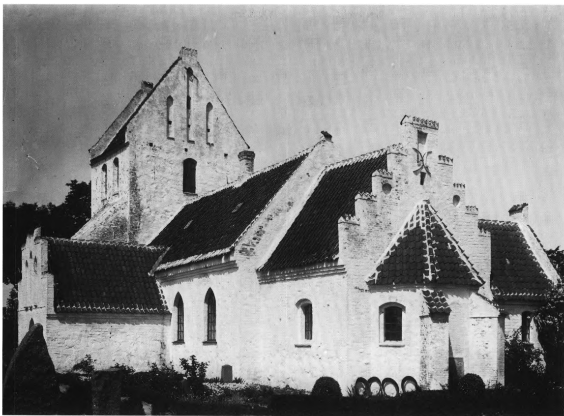
Fig. 5. Ydre, set fra sydøst. Chr. Axel Jensen fot. 1920. - Exterior seen from the south-east.
